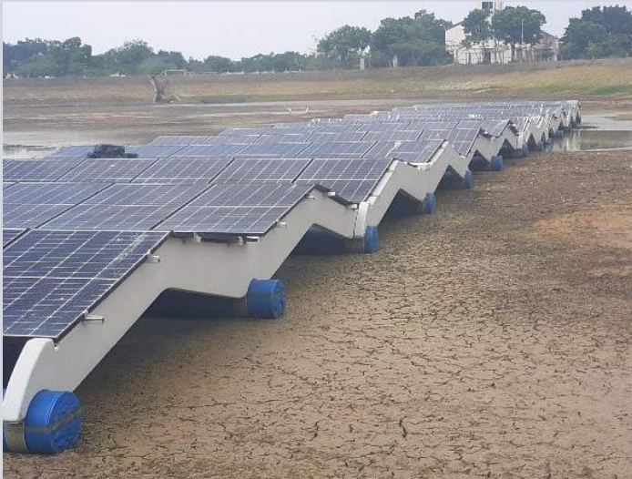
Figure 02 -The floating solar plant during the dry and rainy season
