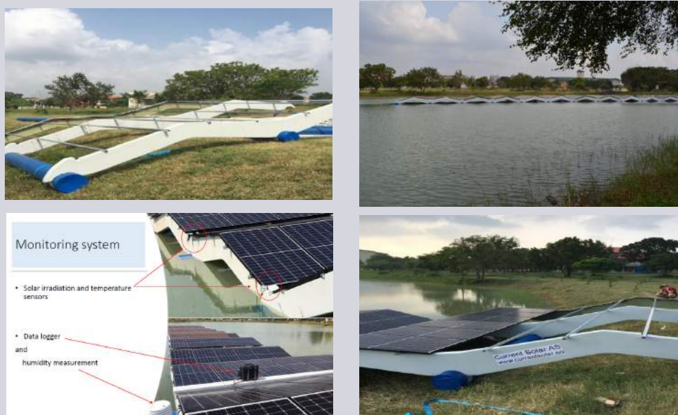
Figure 01: The installation of floating solar plant
